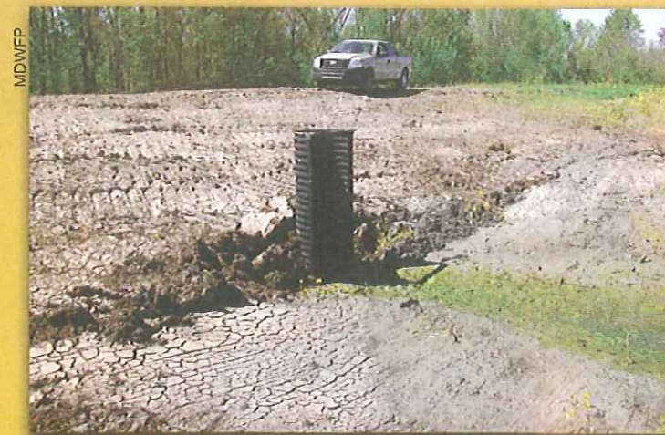
Water control structures like the examples shown above are valuable wetland management tools. Boards are stacked in grooves to allow varying water depths during winter and appropriately timed drainage in the spring and summer.
